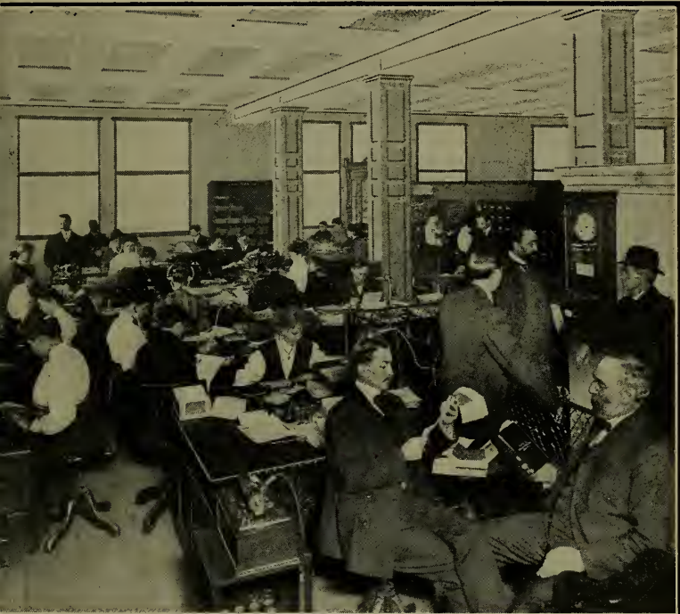
VIEW IN GENERAL OFFICE
